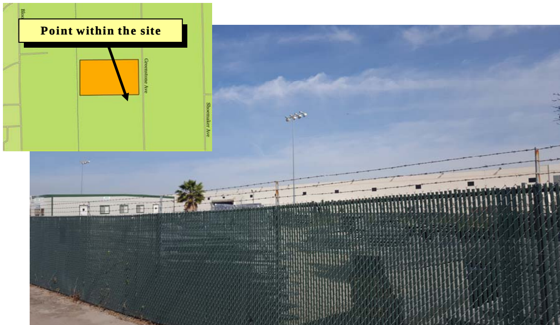
View of interior of project site from southern abutting property line, facing north
