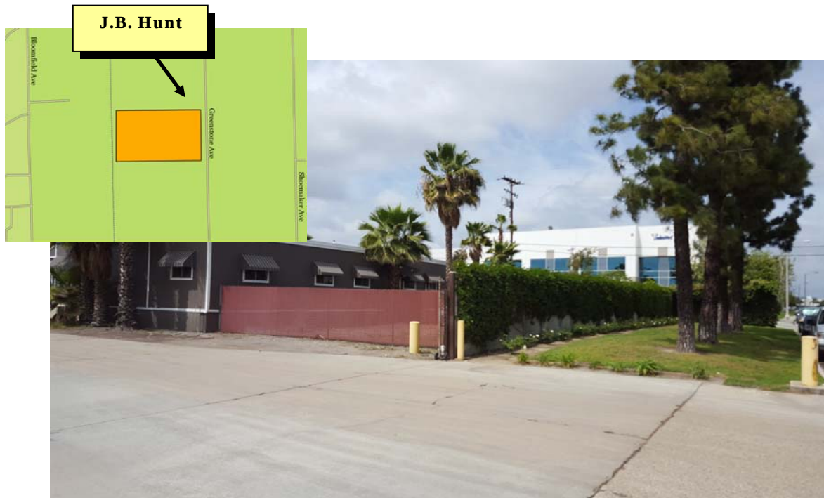
View of J.B. Hunt, north of the project site
