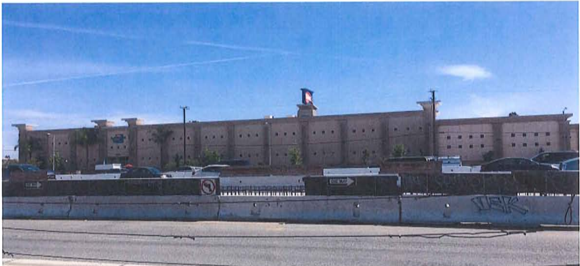
(Close-Up View from east side of 1-5 Freeway)
