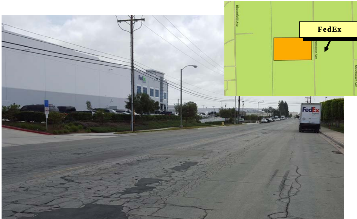
View of FedEx, east of the project site
