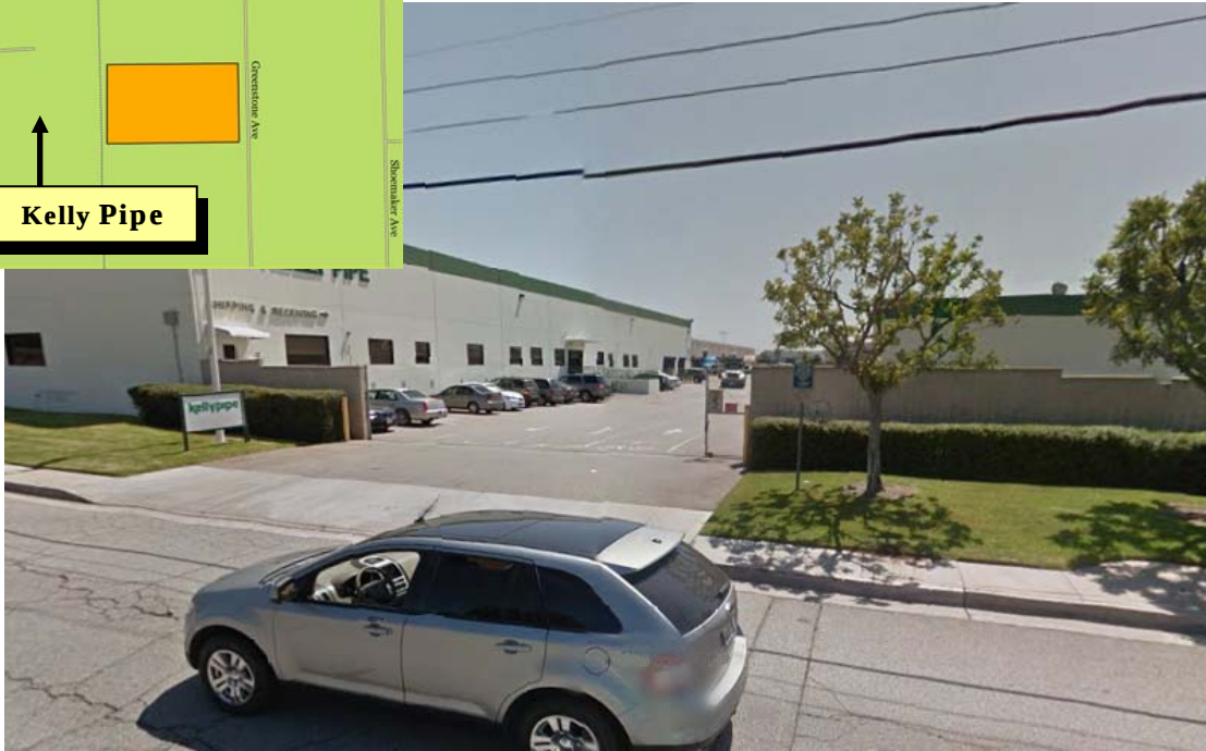
View of Kelly Pipe, west of the project site
